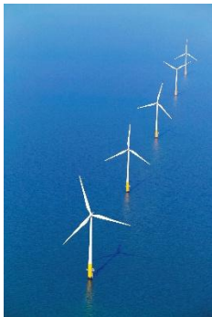
Picture: Copyright Iberdrola
